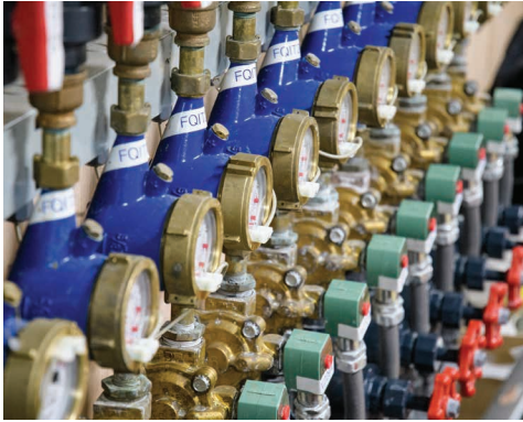
Pumps inject molasses-amended water into groundwater at Garfield Avenue Site.
